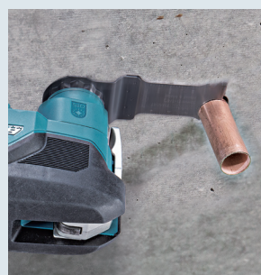
Flush copper pipe cutting
