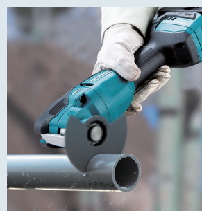
PVC pipe cutting
