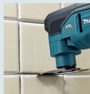
Tile grout removal
