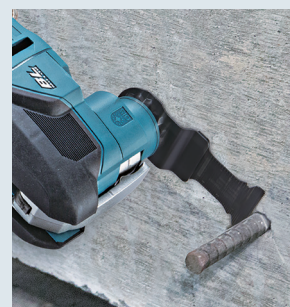
Flush rebar cutting
