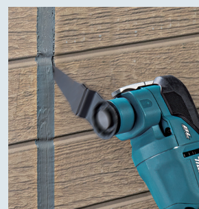
Elastic sealant removal
